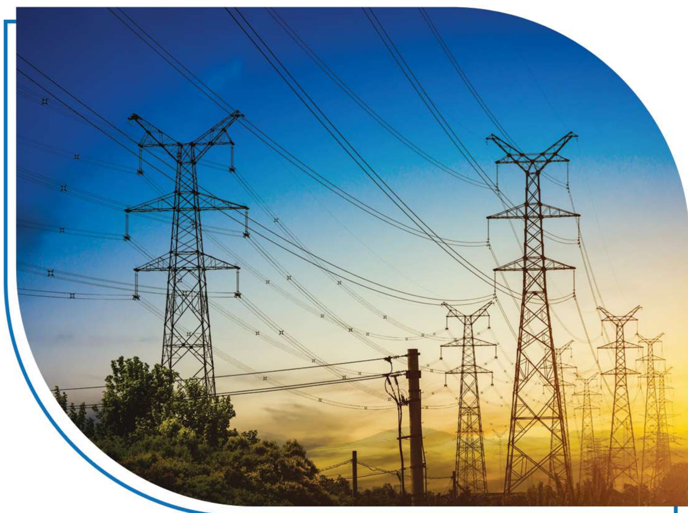
Transmission Line Towers
